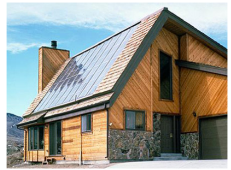
This house is in Golden, CO features a solar water heating system.
